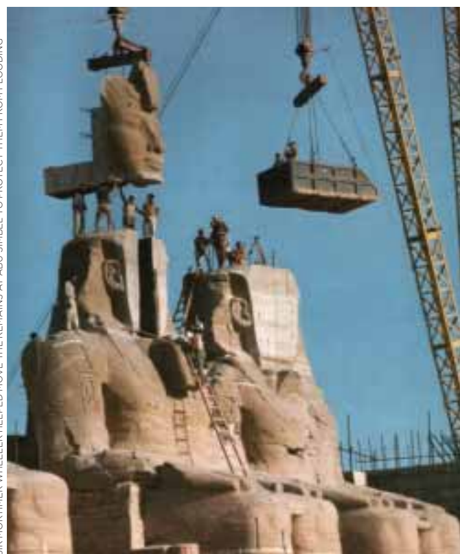
SIR MORTIMER WHEELER HELPED MOVE THE REMAINS AT ABU SIMBEL TO PROTECT THEM FROM FLOODING
